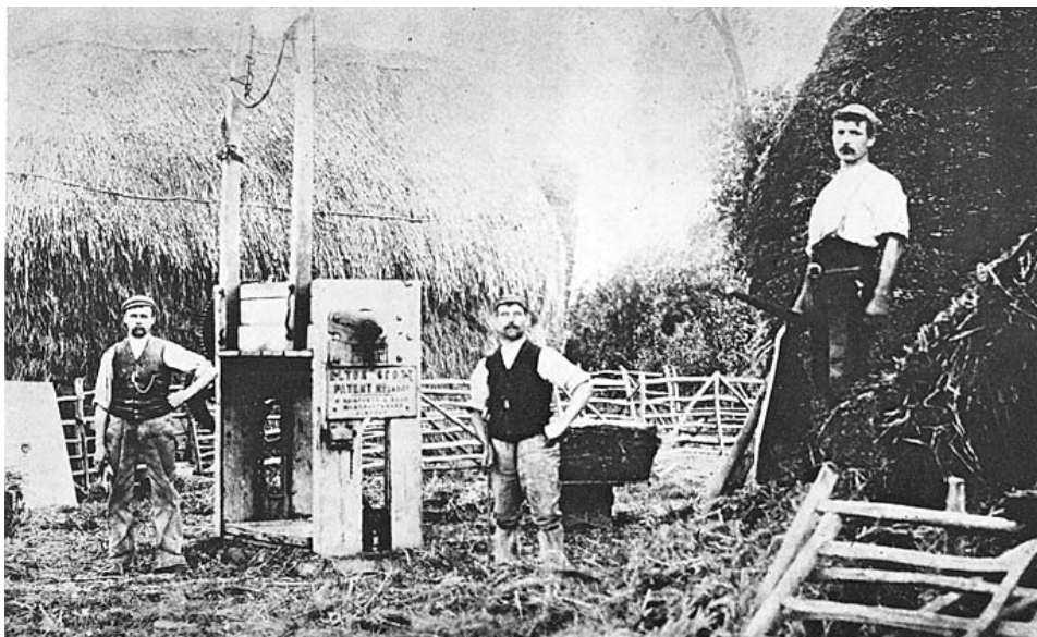
Hay dealers in Norfolk in the early 20th century, would carry hay loose from the field and stack it in their yard. Only later would it be baled in the hand-powered baler pictured above and transported to Norwich for sale. The picture on the right shows a barbed rod used for extracting samples of hay from the centre of stacks. Pictures from George Ewart Evans, The Days That We Have Seen , which has a 30 page chapter on "The Hay Trade".
